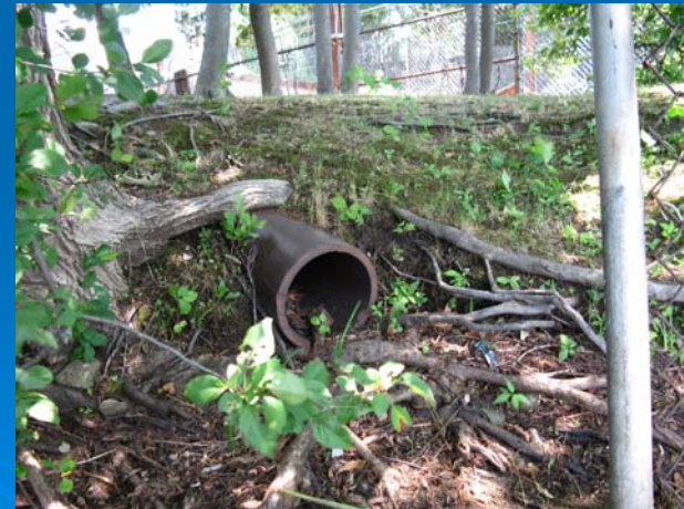
Outfall 4 – no longer in use
