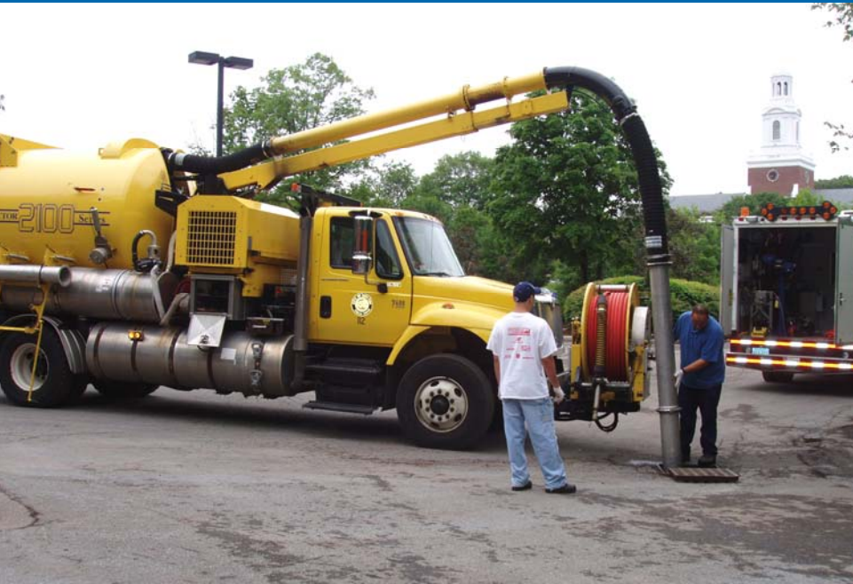
Cleaning drain manholes & catch basins
