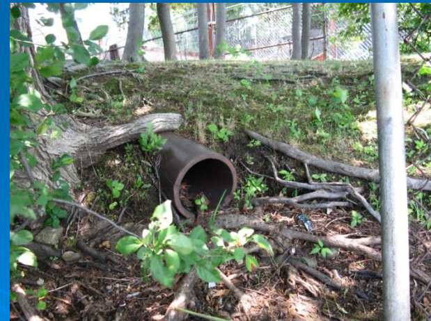
Outfall 4 – no longer in use
